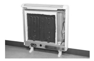
10. Place the heating elements back into their original position. Place the other two rows of storage bricks with the flat side facing out and always on the heating elements supporting tabs.
