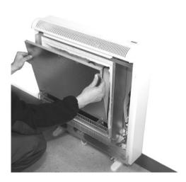
**CAUTION** In the interior part of this inner panel there is a very delicate thermal insulation MICROTHERM panel. It has to be handled with extreme care. AVOID TOUCHING IT.
