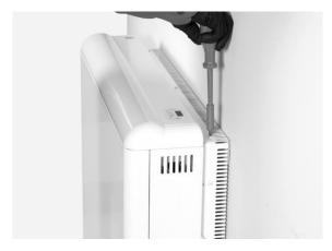
SOLAR HHR MUST NOT BE HUNG ON THE SCREWS; these are used only to prevent the device from overturning and not to support it. If there is any doubt concerning the wall strength, consult the corresponding construction specialist. The appliances are heavy; it is the installer responsibility the correct installation and wall support of these devices to prevent them from overturning.
