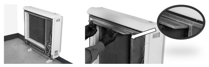
12.- Place the third row of storage bricks with the flat side facing out.
