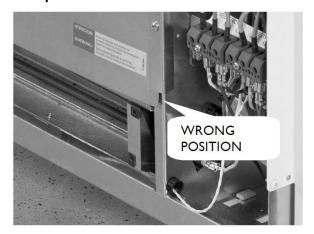
14. Replace the front panel. When refitting the exterior front panel, align the 2 metal upper pegs on the heater with holes in the exterior panel. Push the top up into place and push the bottom in, then refit the screws.
